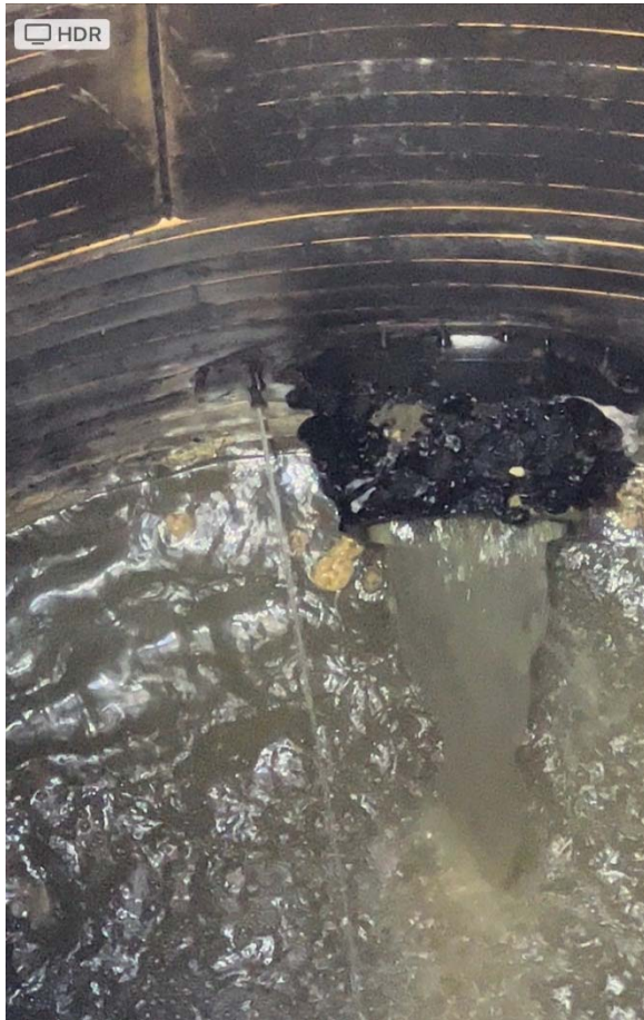
This picture shows the wet-well leak adjacent to the influent pipe. Note stream to the left of influent stream.
